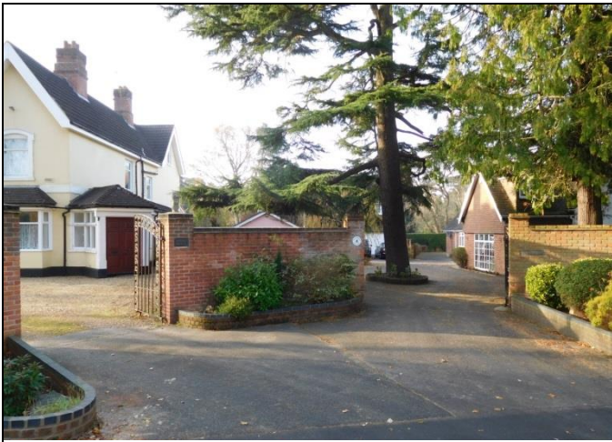
Figure 1F-1 Driveway to Brora House, Nyewood Cottage & Woodlands
