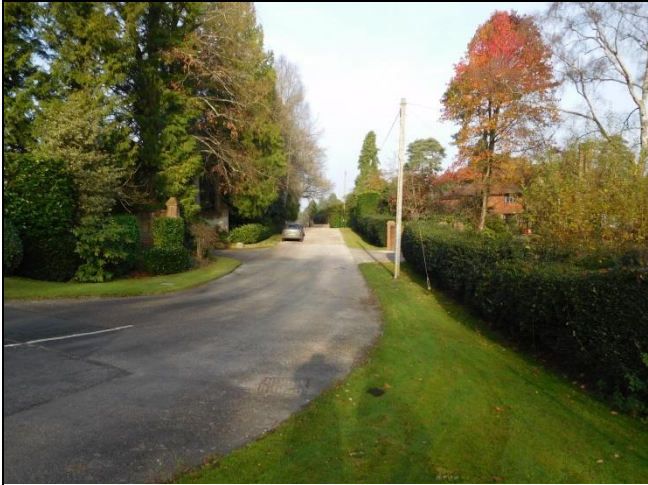
Figure 1C-1 View north on Copse Lane at Chilworth Road end
