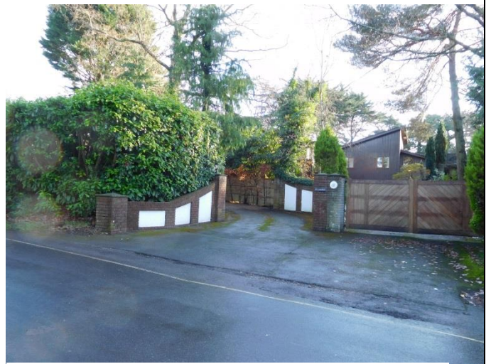
Figure 2D-4 Birch Road, shared entrance
