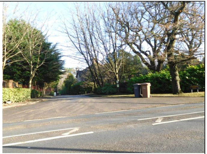
Figure 2B-2 Chilworth Road, south east, shared entrance
